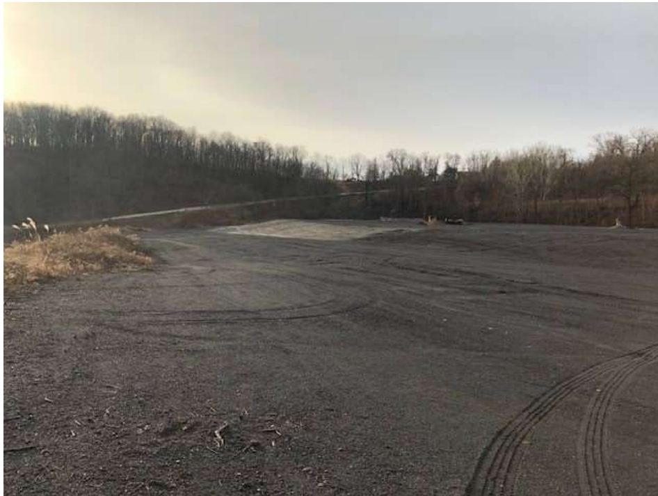
Photograph 8: Southwest view of active area. Material is graded and compacted.
