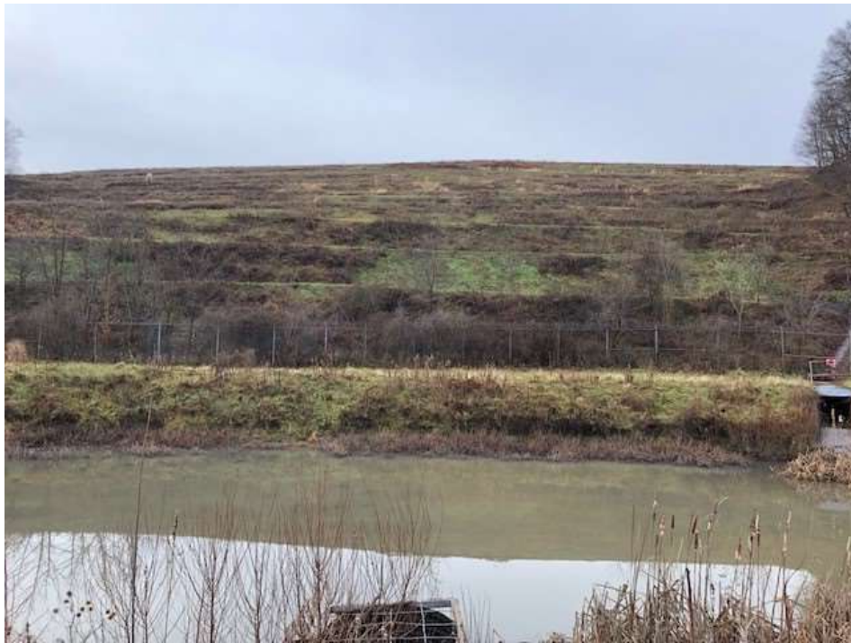
Photograph 17: West view of east landfill slope from Sedimentation Pond spillway.
