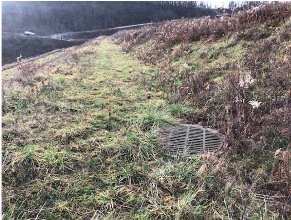
Photograph 9: South view of upper bench and non-contact stormwater inlet on east landfill slope. Vegetation is established with no indications of stability issues.
