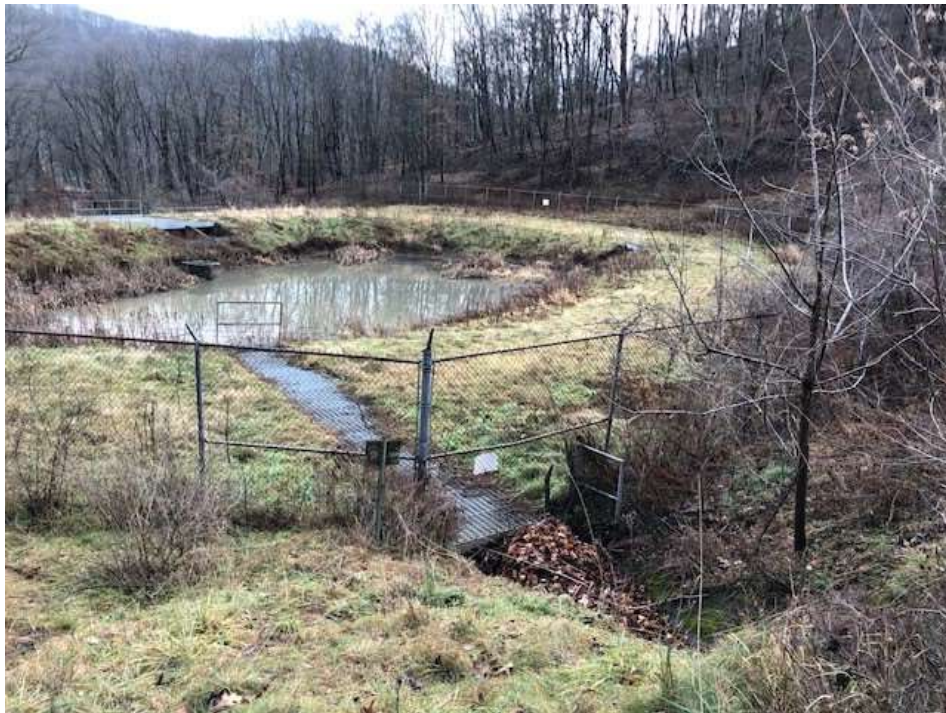
Photograph 16: View of northeast non-contact stormwater inlet to Sedimentation Pond. Some leaves and debris are present, which is regularly removed as needed. Stormwater is flowing freely and is not impeded by the leaves and debris.
