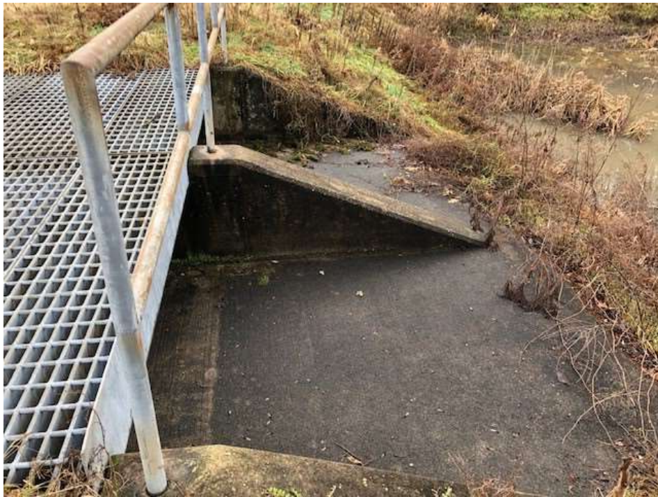
Photograph 19: View of Sedimentation Pond emergency spillway inlet.
