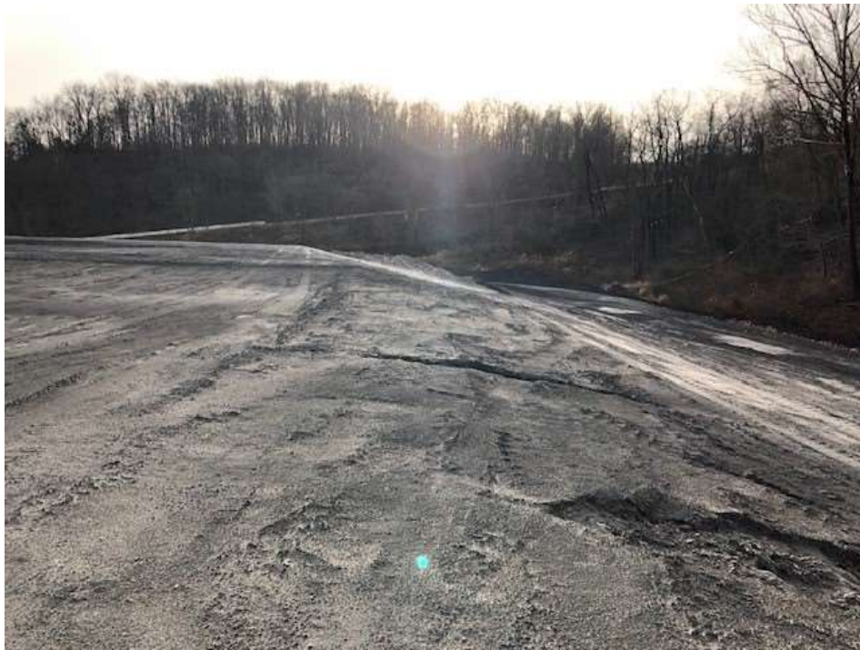
Photograph 5: South view of active area outside west slope. Contact water (leachate) drains to leachate collection layer.
