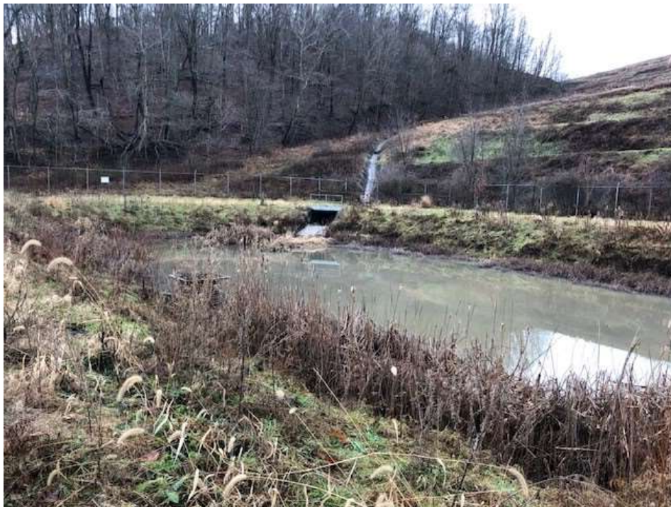
Photograph 18: View of southeast non-contact stormwater inlet to Sedimentation Pond.
