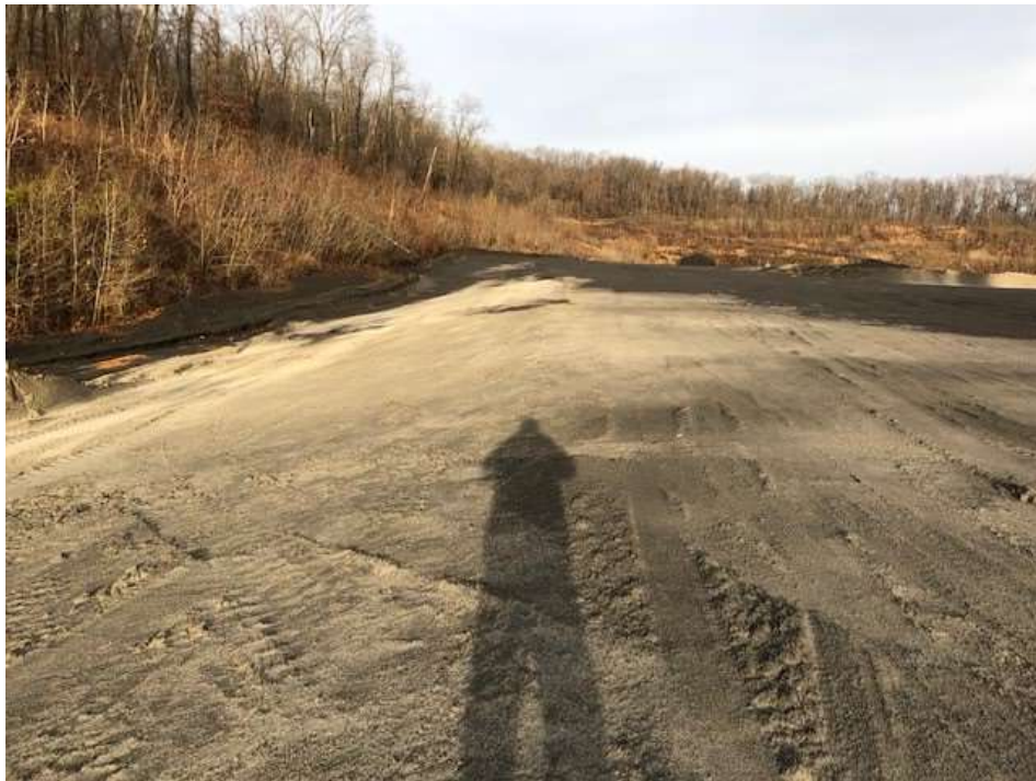
Photograph 6: North view of active area outside west slope. Contact water (leachate) drains to leachate collection layer.
