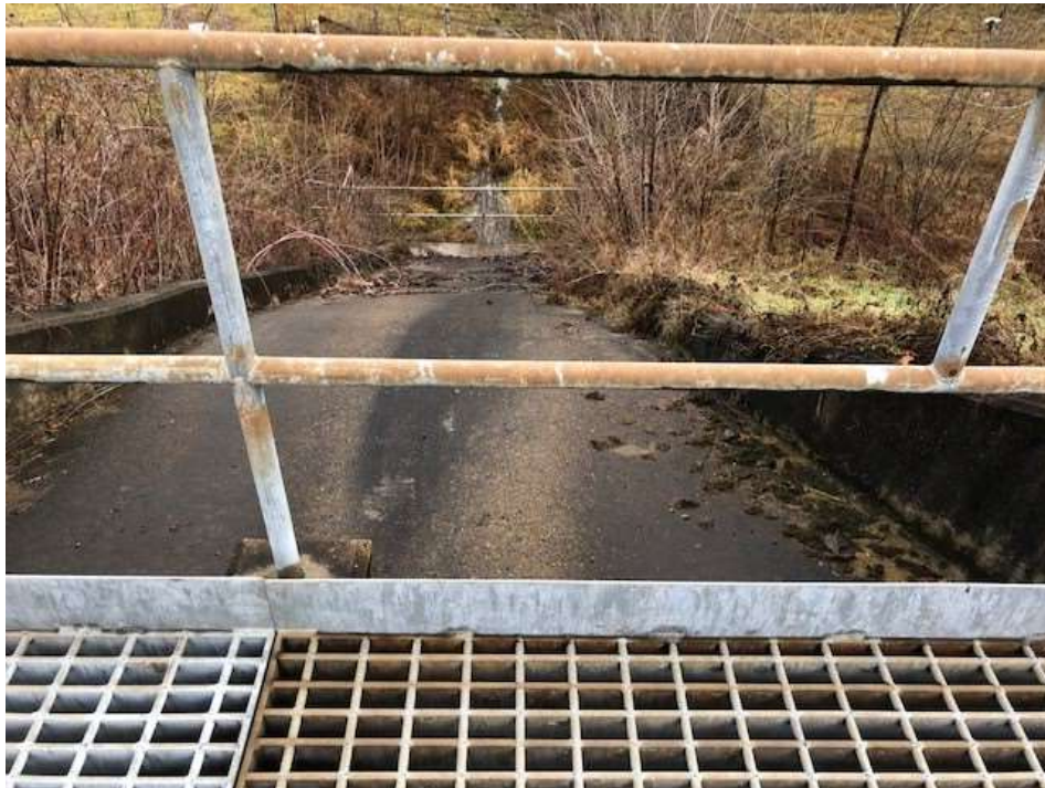
Photograph 20: View of Sedimentation Pond emergency spillway outlet.
