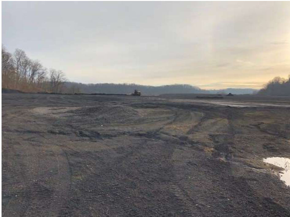
Photograph 2: Eastern view of active area. Material is graded and compacted.
