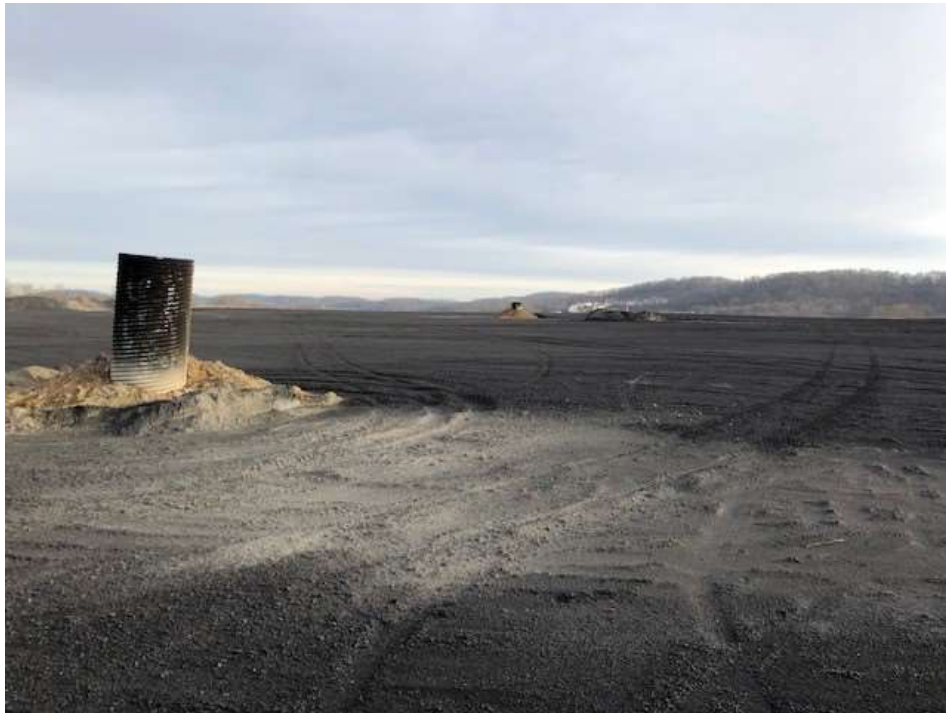
Photograph 4: Eastern view of active area and non-contact stormwater risers.
