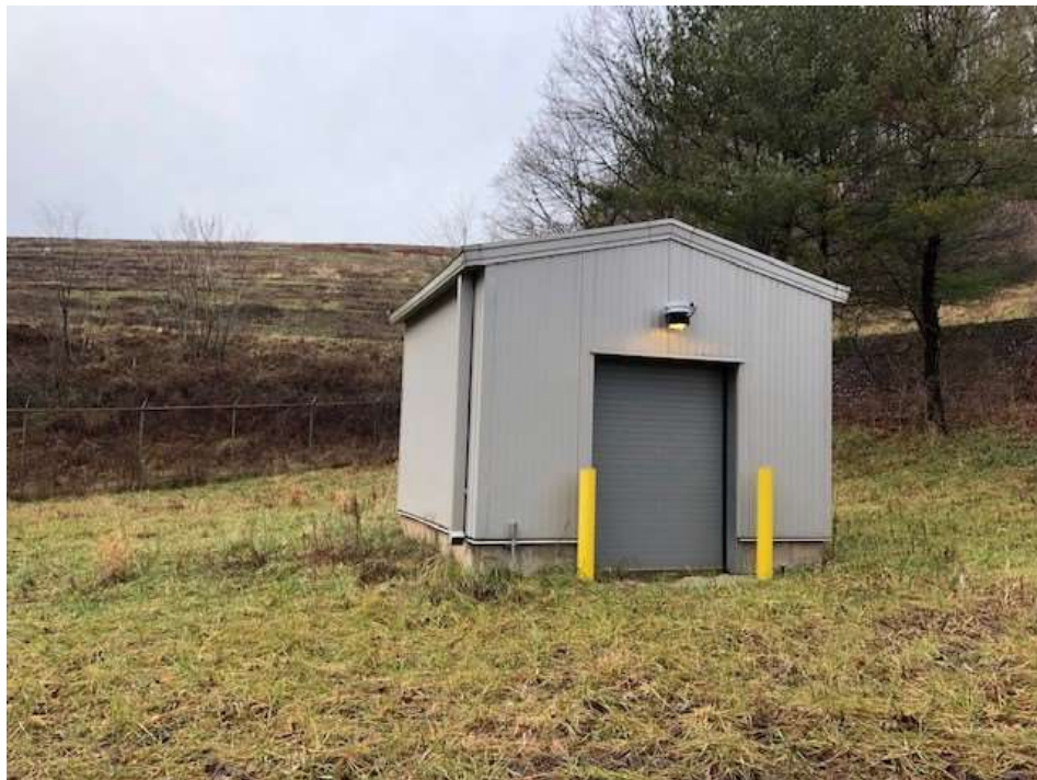
Photograph 22: View of leachate pump station.
