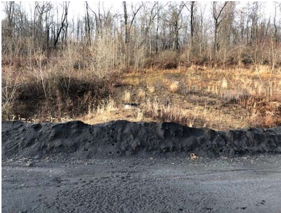
Photograph 3: Non-contact stormwater junction box riser located southwest of landfill.
