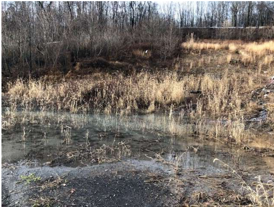
Photograph 1: Non-contact stormwater junction box riser installed in 2020 located northwest of landfill.
